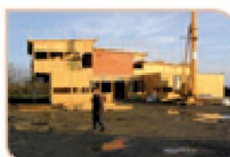
Structure bois (photo Collart)
